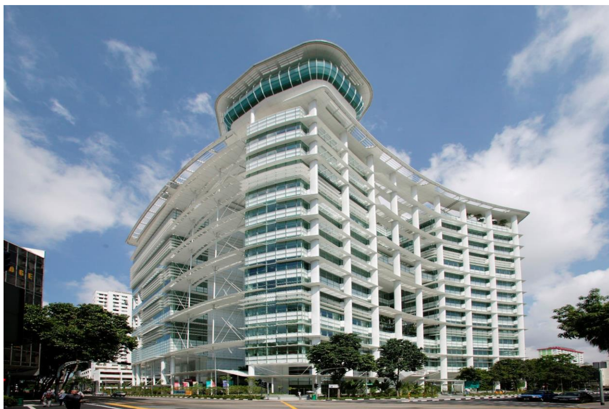
Fig. 1 – National Library Building in Singapore.
